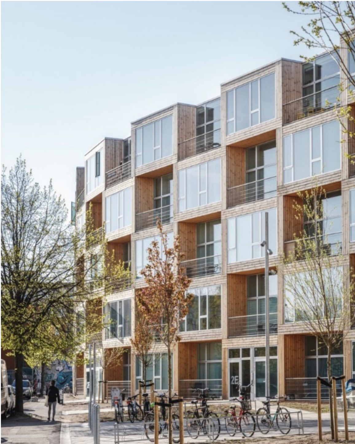
Image 1: Dortheavej development, Denmark
