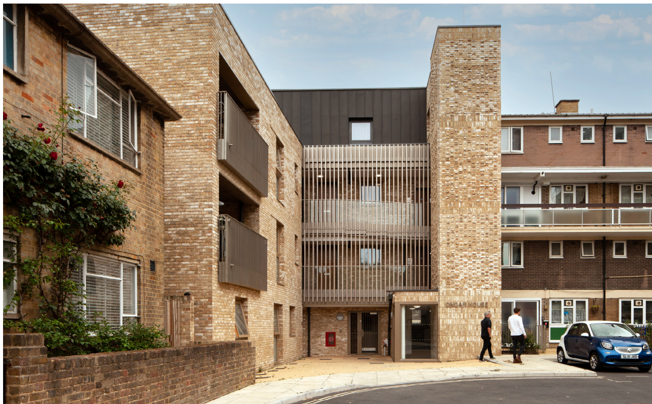
Dover Court Estate. Credit: Pollard Thomas Edwards.
