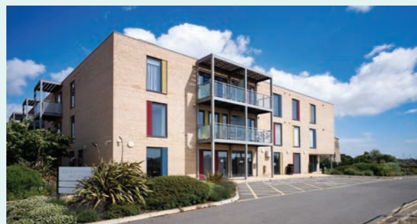
Beaumont House Walton-on-the-Naze, Essex Extra care for over 55s 60 x 1- & 2-bed apartments c.90 people housed
