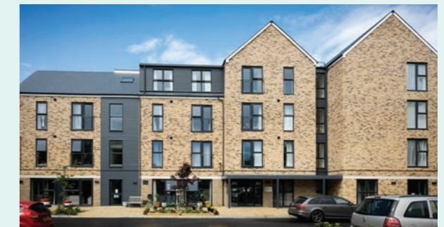
Colwell Road Freshwater, Isle of Wight Extra care apartments, including shared ownership for over 55s, or over 45s with a support need 75 x 1- & 2-bed apartments c.110 people housed
