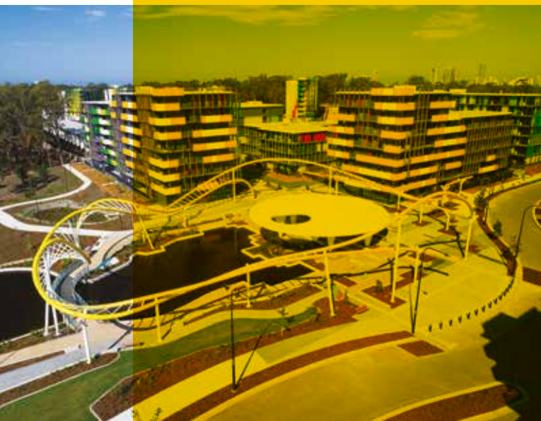
▲ Grocon – Parklands, Gold Coast, Queensland. Australia’s first ‘mainstream market’ build to rent project (re-purposed from its initial use as Commonwealth Games).
