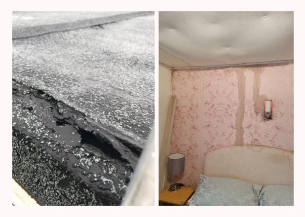
**Left**: The holes in the waterproofing of Mr. Phillips' roof. **Right**: Bowing ceiling from water ingress and damage to bedroom walls and electrics.
