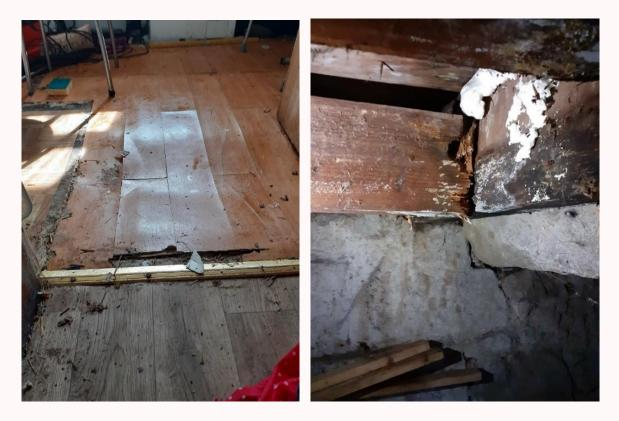
Left: Damaged flooring posing a falls risk for Mr. and Mrs. Howell Right: The rotting support beams in the cellar that threatened to give way. These were supported by Acrow props fitted by Care & Repair.
